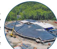
WCMA under construction
