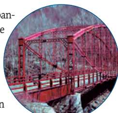
Bardwell's Ferry Bridge
