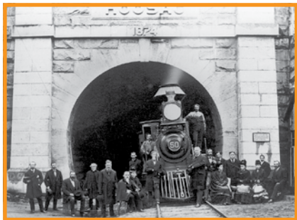
Western Portal of the Hoosac Tunnel NORTH ADAMS
